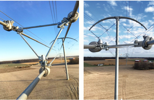
Two types of Loose Spacers used by AEP Copyright © 2025 BOLD® Transmission, LLC. All rights reserved. Used with permission.
